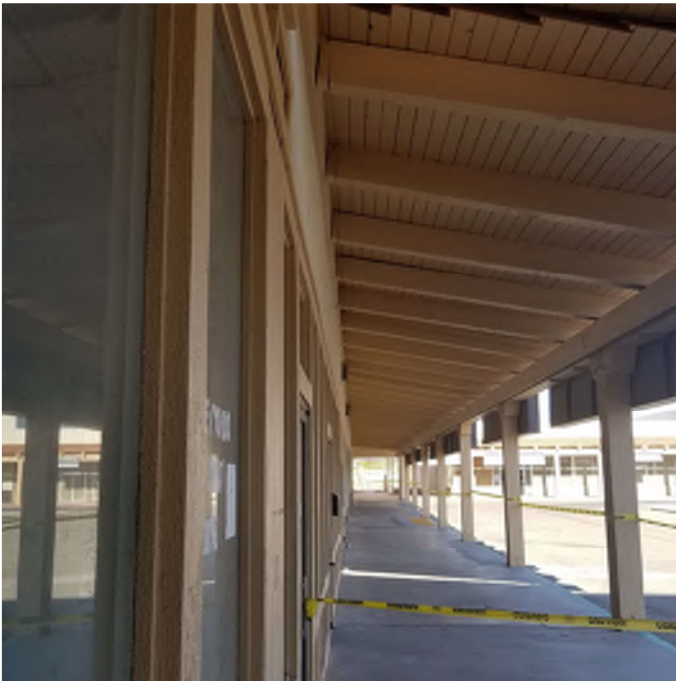
Photo S - Walkway cover
